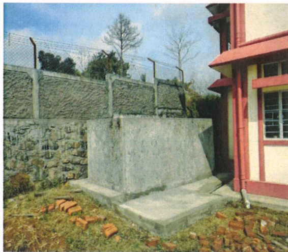
RCC Reservoir (Girls' Hostel)
